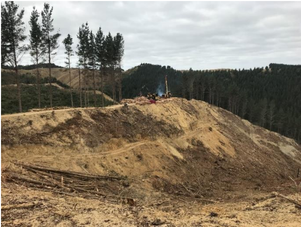
Figure 5 – Poor erosion and sediment controls
