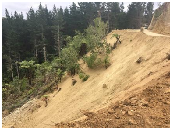
Figure 9 – Side casting of material
